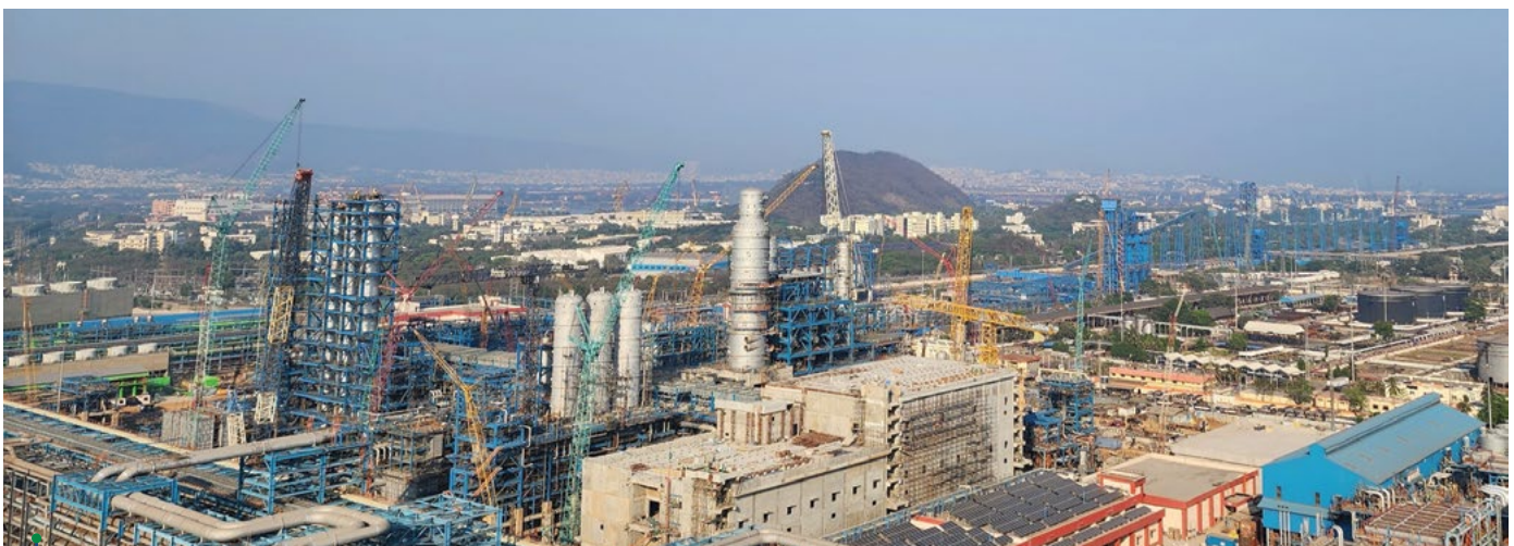
Pioneering progress, transformation unfolds as Visakh Refinery Modernization Project takes shape
